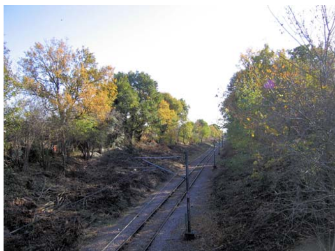
View from footbridge
