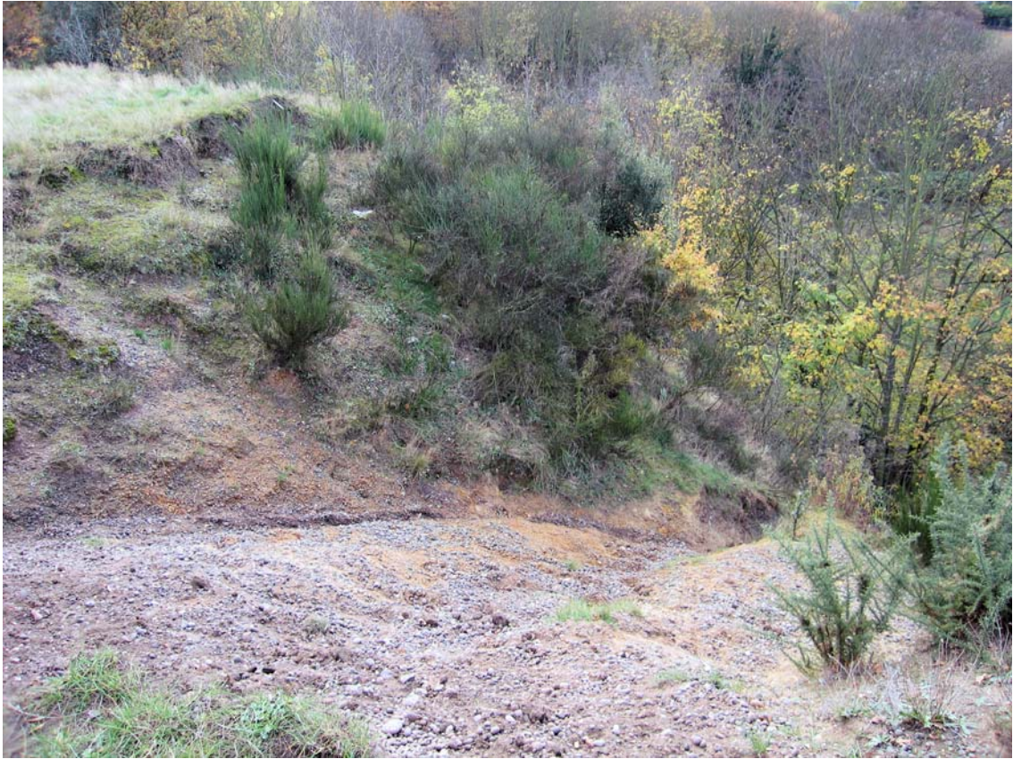
Slumped material viewed from top of site
